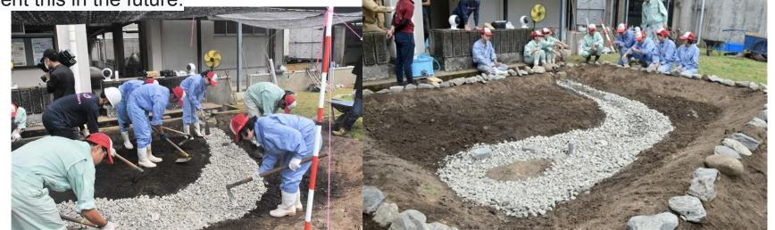
雨庭は、校舎の屋根に降った雨水が雨 どいを通って一気に球磨川に流れ込ま ないよう、いったん地中に浸透させるこ とで治水効果が期待されています。 The rain garden is expected to have a flood control effect by temporarily infiltrating the ground so that the rainwater that falls on the roof of the school building does not flow into the Kuma River at once through the rain gutters.
